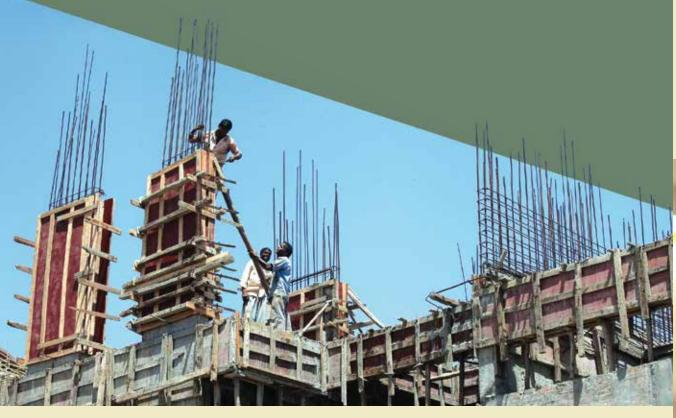
Parameters: Film Faced Shuttering ISI: IS 4990: 1993
